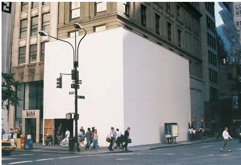
Wall and Scaffolding Installation Corner of 5th Avenue and 53rd Street, New York, NY
