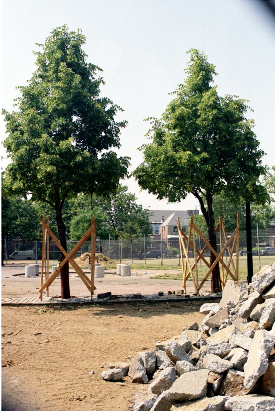
Tree Protectors Installation Brooklyn, NY
